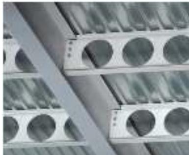
Gambar 3.4 Profil Baja *Circular* (*Castellated and cellular beam*).
